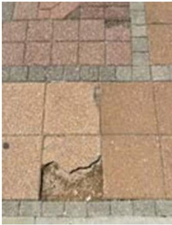
Figure 9 - Cracked Panel
